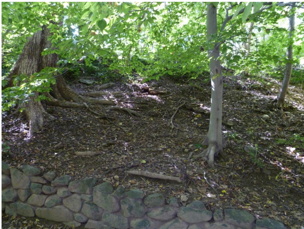
The top photo is a second photo of the same erosional area with vegetation (10-6-2011). The bottom photo shows another eroded slope including the Iris Path stones now visible.
