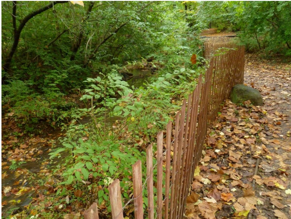
Figure 10: Benefit of Temporary Fencing - These photos taken along the Stream Path show the benefit of temporary fencing for re-vegetation, accumulation of leaves, and slope erosion control.
