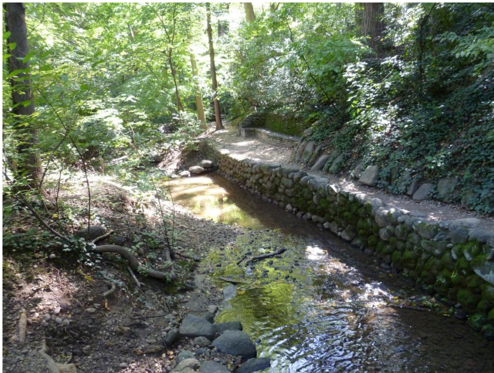
(Above) This photo provides an example of a rock wall near the Stream Arbor designed by Beatrix Jones Farrand to protect soils and Stream Path from high stream velocities. The 30" headwaters pipe is shown below. (10-6-2011 photos)
