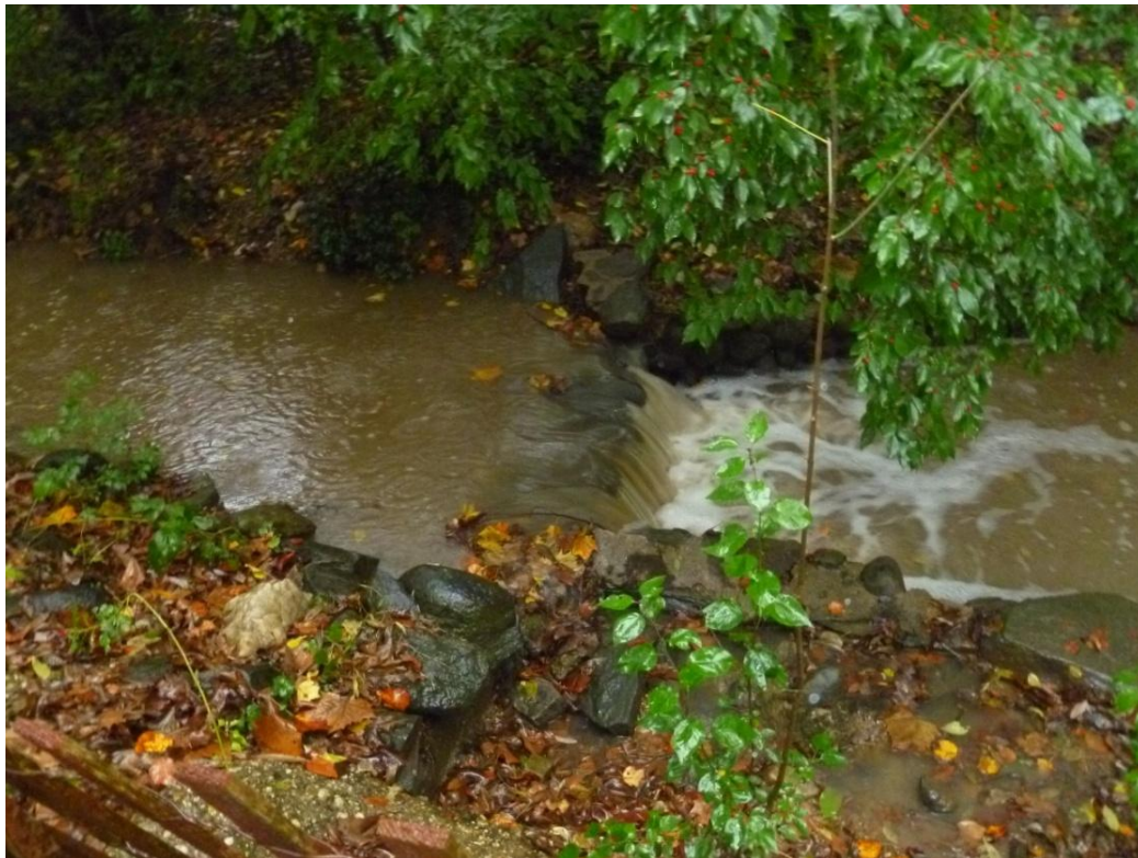
Three Bridge Falls (E) at 10:01A – water volume exceeds the capacity on the south side of the structure.
